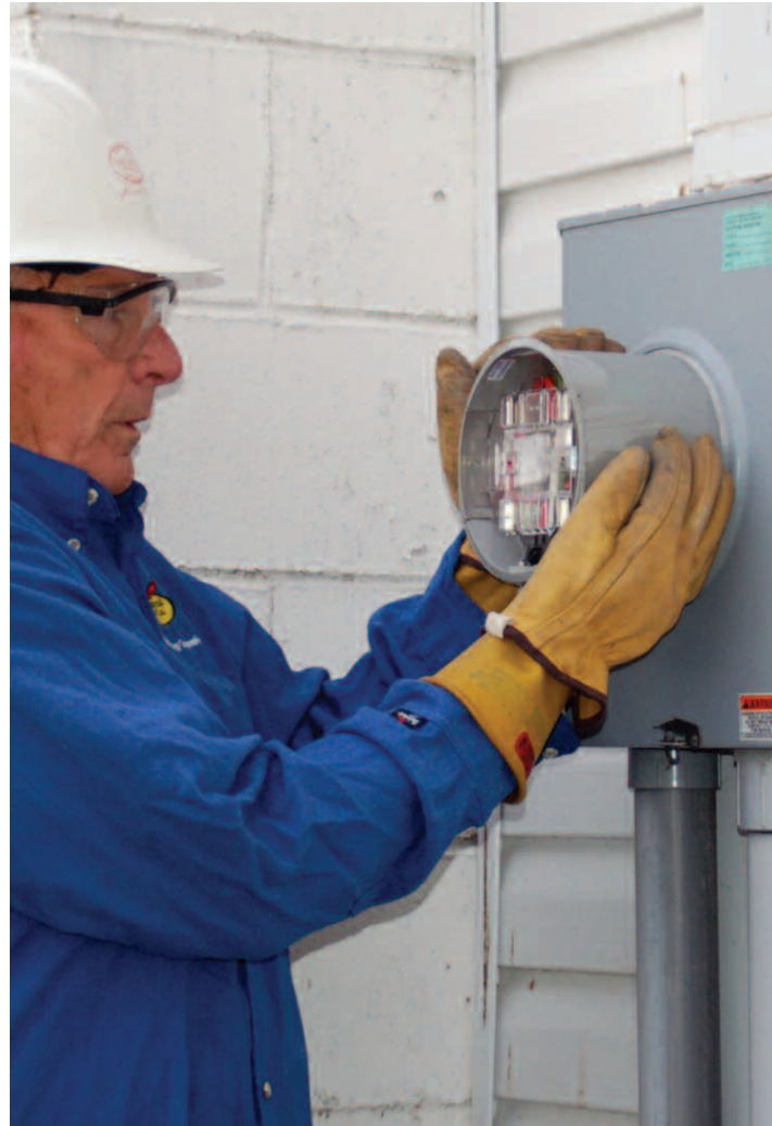
Meter Technician Jack Bitler installs a GenerLink unit for a customer.
